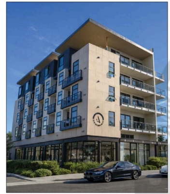
Elda Developments is finishing construction of a micro-apartment building in Normal Heights. Photo courtesy of Elda Developments
